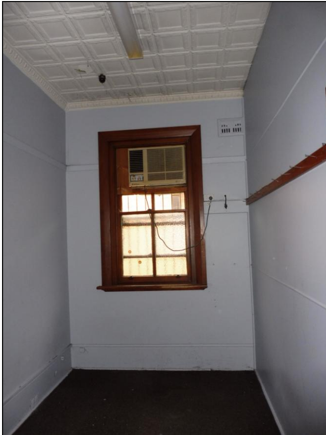
Figure 3.51 Lightweight partitions have been added to divide the former recreation space into two spaces with an access hall. The space retains the high, pressed metal ceiling and cornices, some rendered walls details, windows and high wall vents on the external wall.
