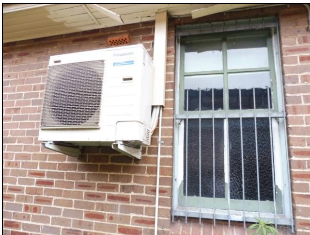
Figure 3.36 Detail of one of the southern side windows. Note the AC unit and damage to the boarded eaves lining.
