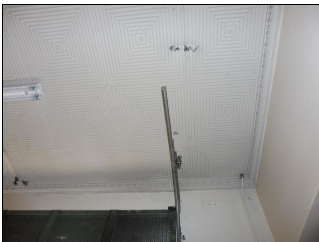
Figure 3.39 The pressed metal ceiling over the engine bay has a diamond pattern with egg and dart pressed metal cornice. The ceiling is in good condition, however, some penetrations have been made and services added.
