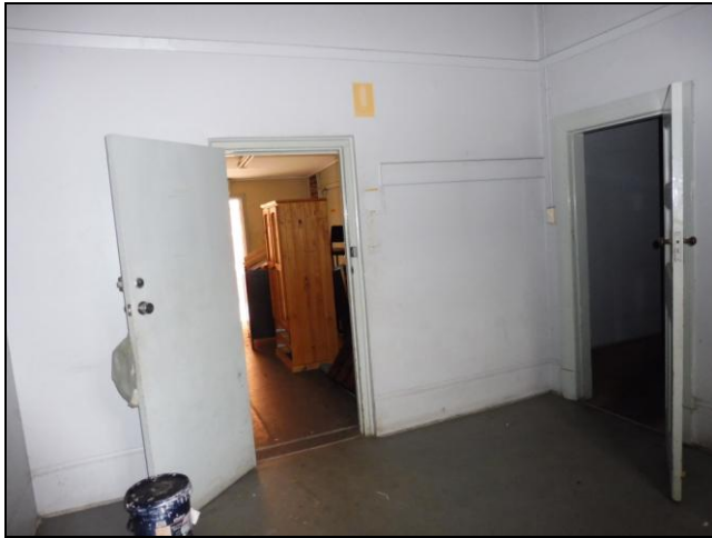
Figure 3.59 The original single men's room has been converted into a kitchen. The original door and access from the main wing remains (at right). The original north facing window appears to have been converted into a door (at left) and connects to the c. 1997 addition
