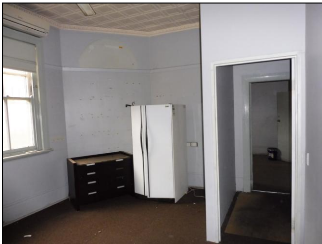
Figure 3.54 The former recreation space retains a splayed fireplace breast, high pressed metal ceiling and original windows on the external (southern) wall.
