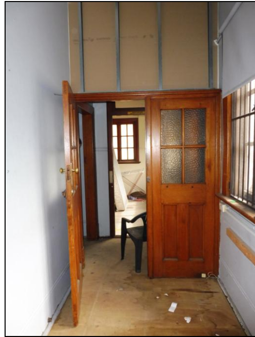
Figure 3.48 The former watch room also retains rendered skirting and details on the external wall, timber windows (overlooking William Street) and architraves with the original stain finish, wall vents and high pressed metal ceiling. Surface mounted services have generally been added.
