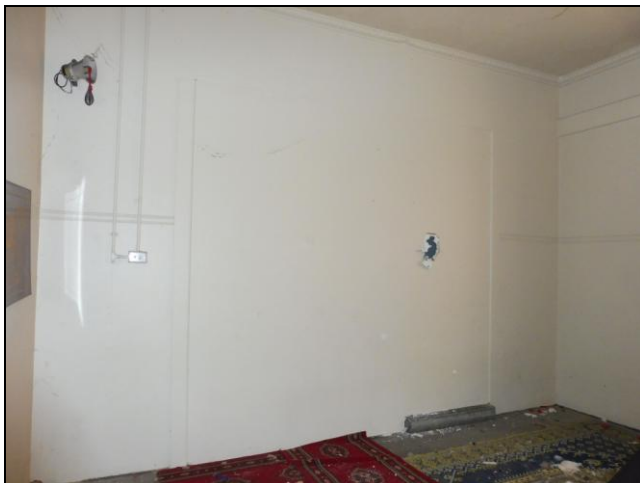
Figure 3.46 Lightweight (plasterboard) infill has been fixed to the internal face of the original wide opening on the western wall of the former engine bay. The original doors are visible on other side of the wall. Two of the three original doors remain.
