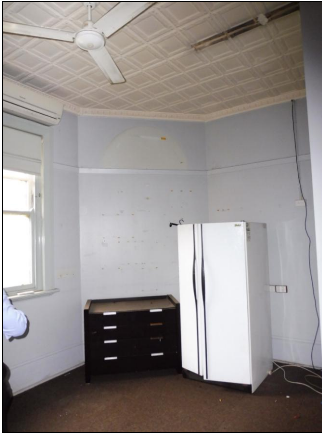
Figure 3.56 The splayed fireplace breast. The fireplace has been infilled and surround has been removed.
