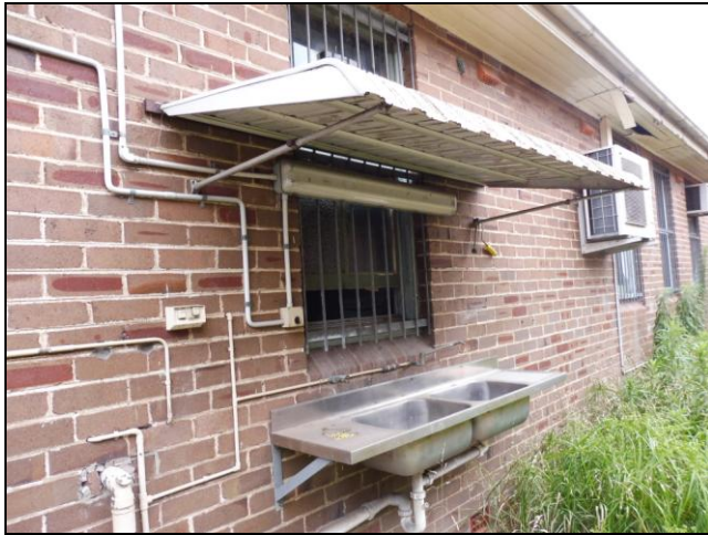
Figure 3.35 The southern façade and part of the eaves lining has been affected by the addition of services including a sink, lighting and air conditioning units. A modern steel bracketed awning has also been fixed to the façade.
