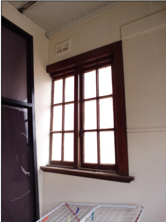
Figure 3.40 The former engine bay retains two sets of 6-paned timber framed casement windows and architrave with the original stained timber and varnish finish. The walls also have inscribed dado rail, picture rail and high, decorative wall vents.
