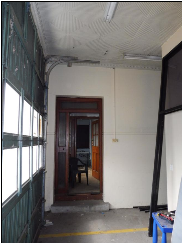
Figure 3.41 An opening with original timber frame, top and side light is located in the south eastern corner of the former engine bay. The engine bay concrete slab floor is at a lower level than the adjacent timber floor.
