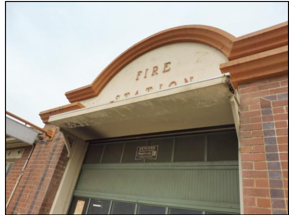
Figure 3.11 The front façade comprises of two bays. The northern bay retains wide opening which was modified as part of the c. 1997 work, but retains the original wide brick piers. The hood was also replaced a modern panel door has also been added to the opening as part of the c. 1997 works to the building.
