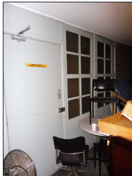
Figure 3.46 Lightweight (plasterboard) infill has been fixed to the internal face of the original wide opening on the western wall of the former engine bay. The original doors are visible on other side of the wall. Two of the three original doors remain.
