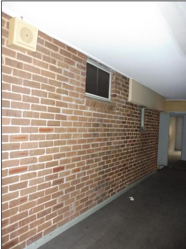
Figure 3.27 Differing brickwork further along the northern façade of the rear wing and bulkhead occurs in line with what is assumed to be an early, skillion roofed addition. The bulkhead/ infill is assumed to have been added as part of the c. 1997 works.
