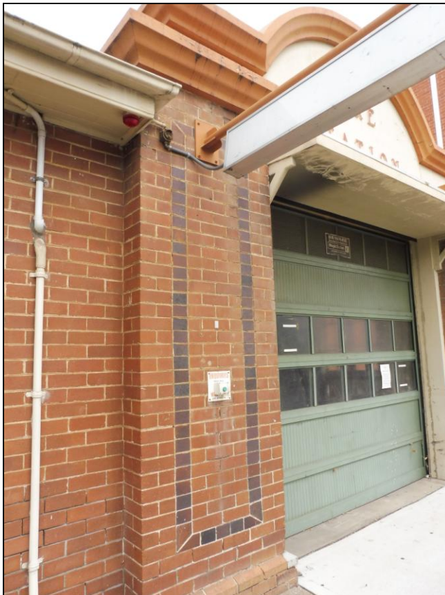
Figure 3.12 Service elements including the emergency call button and signs have been added (and removed) from the façade. The brickwork at the base of the central pilaster has sustained some damage. Some of the mortar joints in the brickwork have also failed.
