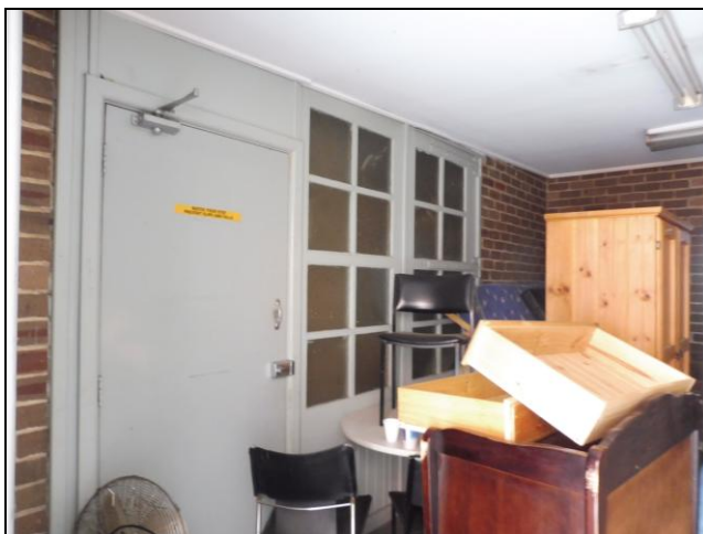
Figure 3.23 The former rear wall of the main wing which was internalised by the c. 1997 additions. The wide former engine room rear opening remains, however, the original timber doors have been modified.
