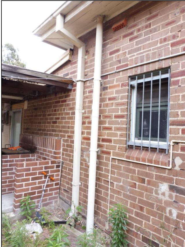
Figure 3.33 The brickwork at the southern façade has no signs of additions, however some variation in the bond is evident. The original plan shows a “drill tank” at the end of the rear wing which may have been enclosed by a brick wall. In 1938, by which time it is assumed that the brick skillion roofed section is assumed to have been added, the tank was shown in the location of the B-B-Q.
