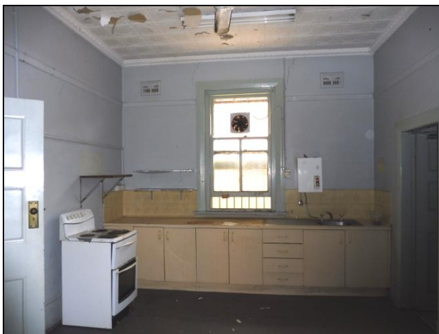
Figure 3.60 The former single men's room retains a high pressed metal ceiling and cornice, high wall vents and window on the external (southern) wall. The original door to the bathroom remains (at right).
