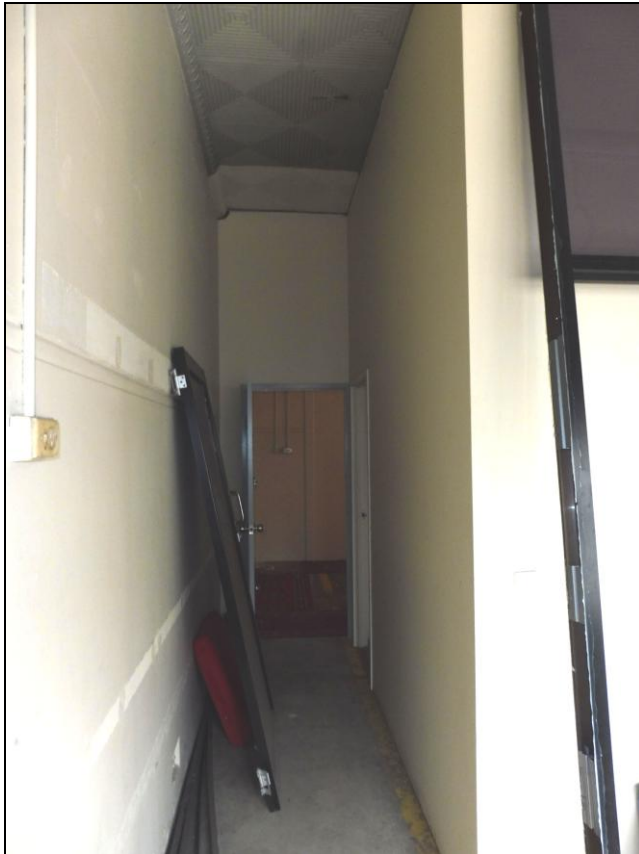
Figure 3.42 Lightweight partitions and reproduction doors have recently been added to create separate rooms in the former engine bay. The southern wall retains evidence of a former coat rail.
