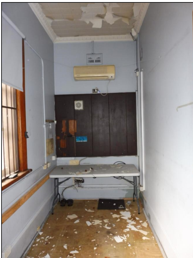
Figure 3.48 The former watch room also retains rendered skirting and details on the external wall, timber windows (overlooking William Street) and architraves with the original stain finish, wall vents and high pressed metal ceiling. Surface mounted services have generally been added.
