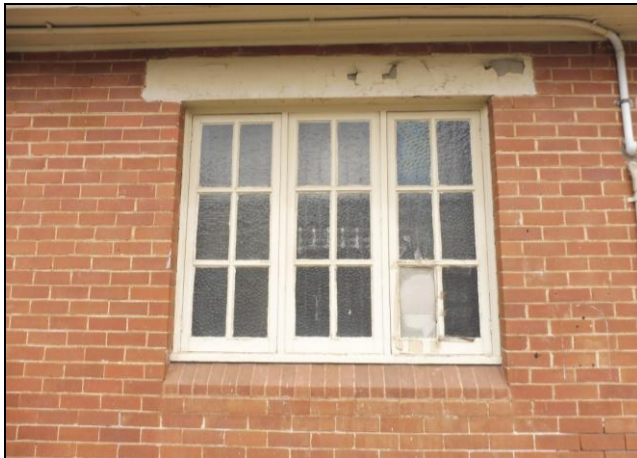
Figure 3.14 The timber framed fixed and casement windows on the front, William Street façade.
