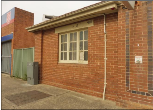
Figure 3.13 The southern bay which has a set of timber framed windows with a simple brick sill and painted lintel over.
