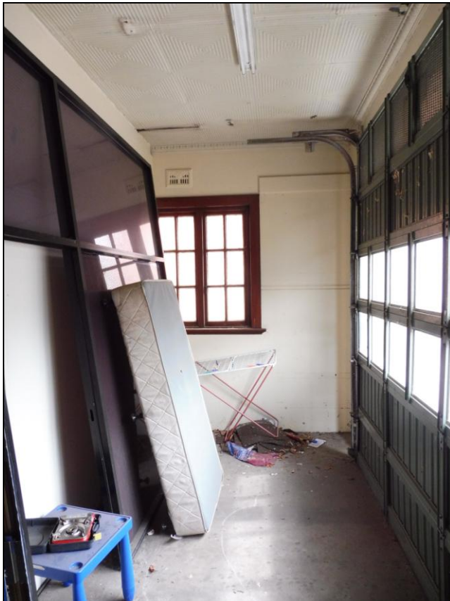
Figure 3.38 The former engine bay which has concrete floor and high pressed metal ceiling and cornice. The original timber doors have been replaced with a model panel door. An inscription in the rendered surround indicates that work was also undertaken to this area in 1997.
