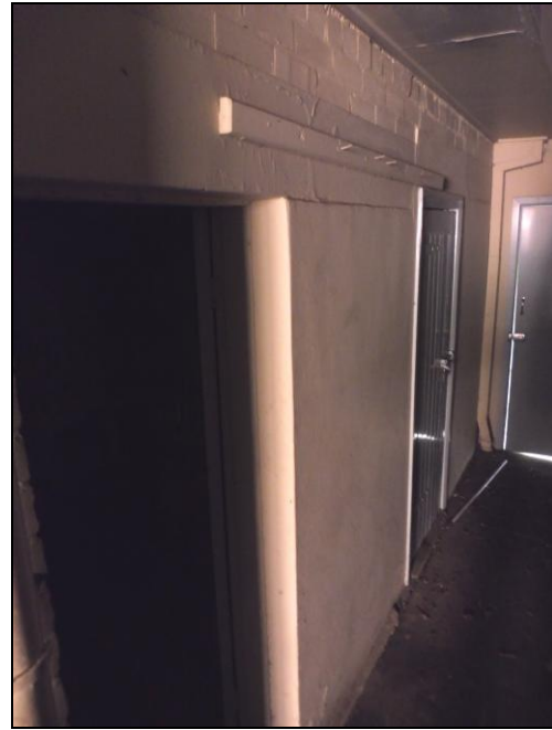
Figure 3.64 Two simply finished store rooms are located at the western end of the rear wing. Assumed to have been early additions they were originally externally accessed. The original rear wall (at left) has been rendered.
