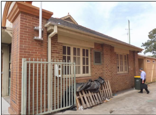
Figure 3.18 The northern façade of the main wing of the building also comprises of two bays divided by projecting pilaster. A gate post and flag pole been added to the north eastern corner (c. 1997). A vented opening also appears to have been added at this time.
