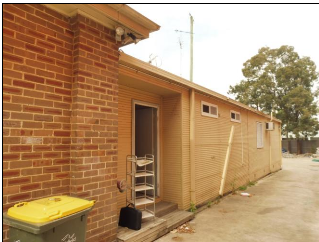
Figure 3.22 The lightweight rear wing addition which is clad in timber boarding and metal sheeting.
