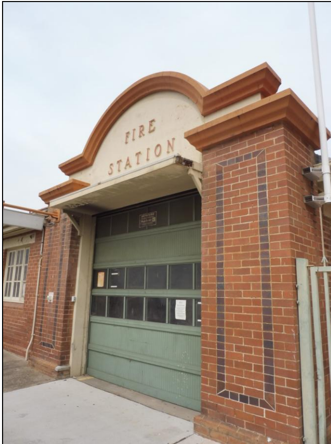
Figure 3.11 The front façade comprises of two bays. The northern bay retains wide opening which was modified as part of the c. 1997 work, but retains the original wide brick piers. The hood was also replaced a modern panel door has also been added to the opening as part of the c. 1997 works to the building.
